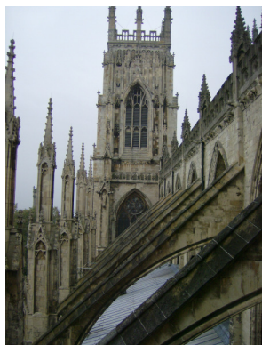
A view of the buttresses that adorn the York Minster
